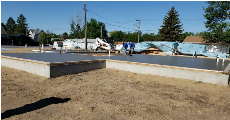
Nelson Concrete putting final touches on the concrete slab of our current twin home.
